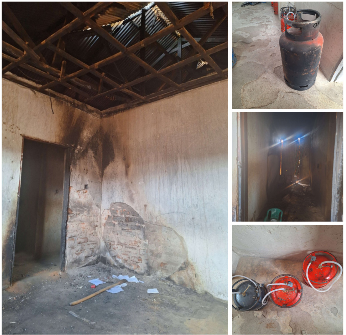
Figure 49: A fire incident related to illegal refilling of LPG Cylinders at Kagomu Street, Mahina Ward, Mwanza City in Mwanza Region
